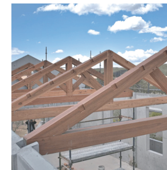
Wood Truss Roof
